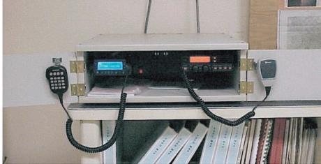
thing that came out of the Indian Fire in 2002 was the lag time in communications between the Fire Center and the Yavapai County Emergency Operating Center (EOC). This installation gives direct radio contact between the two and it was activated two times this past year.
